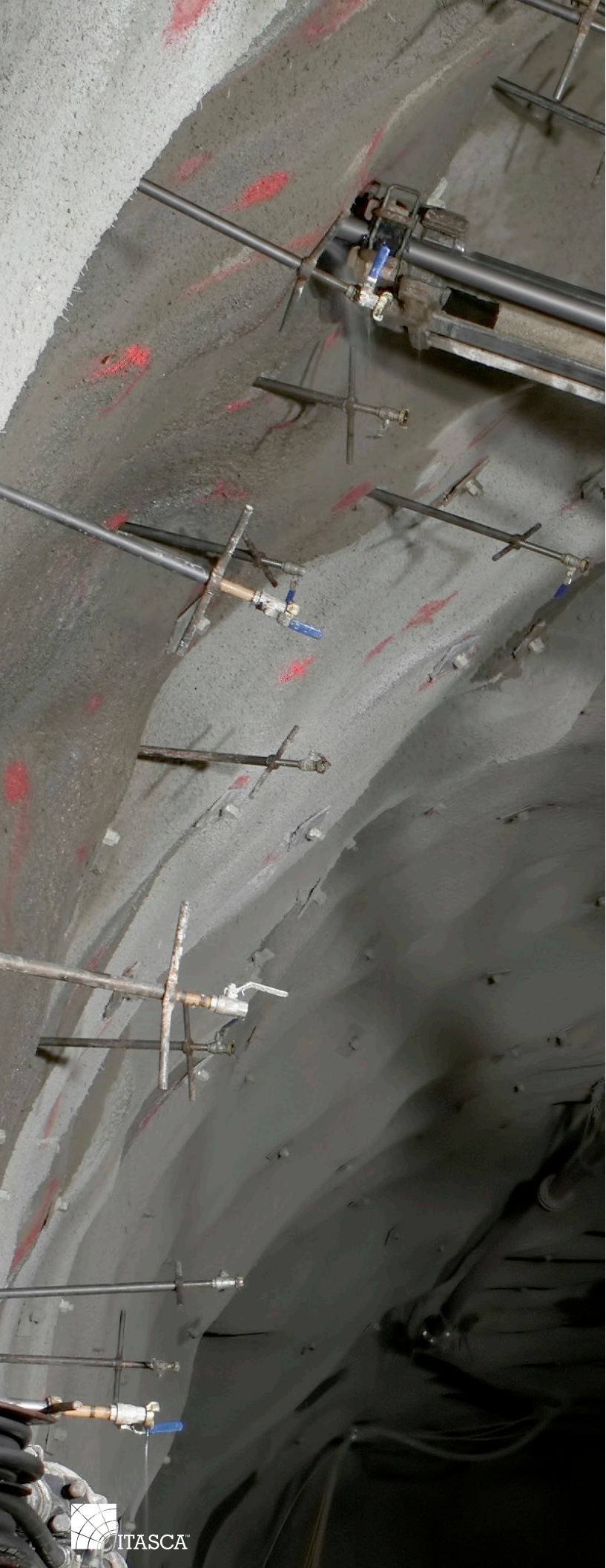
Evaluation of an underground cable bolt and shotcrete support design using FLAC3D . Loads acting axially along the cables are indicated.
